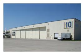
End User: Hangar 10 Location: Kansas City, MO Facility: 25,000 sq. ft. hangar Opening: 197' wide x 28' high Configuration: Six-leaf, full-left and full-right floating door system on six continuous tracks Features:
