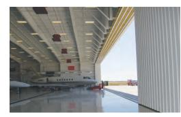
End User: Hawker Beechcraft Services Location: Indianapolis, IN Facility: 40,000 sq. ft. maintenance hangar Opening: 252' wide x 28' high Door Configuration: Four-leaf floating door system on four continuous tracks Features:
