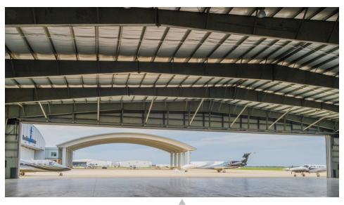
of hot-rolled steel. All members are predrilled utilizing computer controlled fabrication for easy bolt-together installation.
