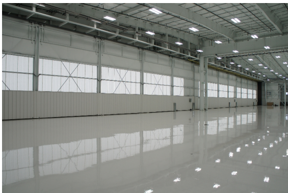
Aero Colorado Hangar - Centennial, CO
